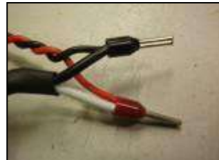
Twist the red wire with the white wire and then the two black wires together as shown and crimp with red and black 1.5mm bootlace ferrules as shown
