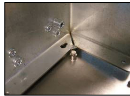
2) Align mounting hole with standoff
